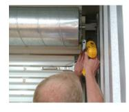
Line the hole on the brackets up with the holes left in the jamb. Secure the Janus bracket to the wall using appropriate fasteners supplied. Repeat this step on the other bracket.
